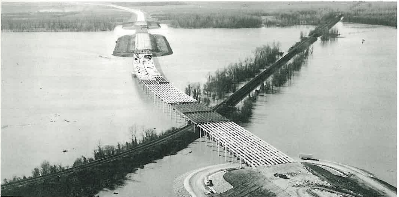
Mississippi flood waters back up toward the levee (arrow) and rise menacingly under the elevated section of I-40 from the Arkansas end of the bridge, westward over the StL & SF Railroad and on toward West Memphis (top of picture). Decking is being put down by the contractor, Holloway Construction Company of Wixom, Mich. The project is being handled by the Tennessee Highway Department.
